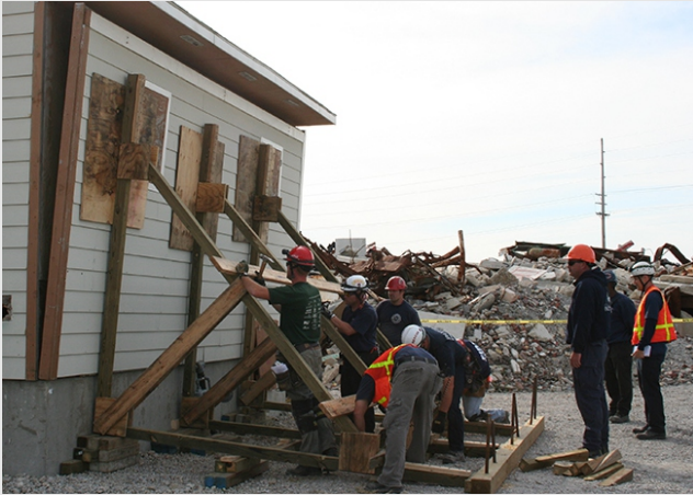
The Illinois Fire Service Institute "Rescue City" included a series of debris pile training props that simulate structural collapses. Students in the Structural Collapse Technician course learn how to operate at an event involving the failure of a building constructed of steel, concrete, or masonry, and practice techniques for cutting, breaching, lifting, stabilizing, searching, shoring, packaging, and removing victims from the simulated collapse environment.
