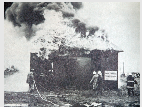
During the 33 rd Illinois Fire College in 1957, two identical houses were burned but extinguished differently for a demonstration comparing straight stream and fog stream firefighting techniques. The demonstration was held on North McKinley Avenue in Champaign.
