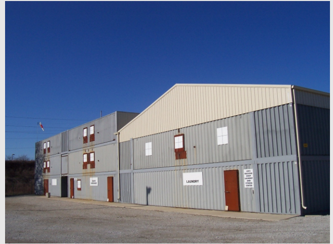
The IFSI Streetscape training prop is one of many simulated structures that allow firefighters to develop skills tailored to specific firefighting environments.
