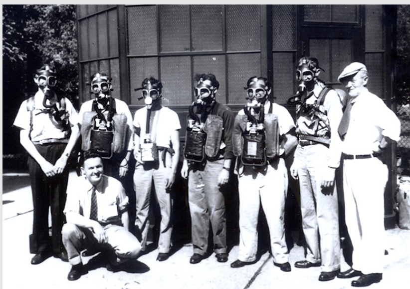
The 8th Illinois Fire College introduced gas mask training, prompting the University of Illinois to construct a smoke building for gas mask training during the 1930s. Like the first permanent training tower, the smoke building was demolished in 1958.
