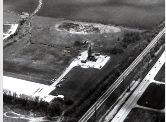
In 1965, the Illinois Department of Public Safety allocated $125,000 from the state's Fire Prevention Fund to construct a six-story fire training tower near South First Street in Champaign. The University had purchased the land in 1961, setting aside twenty-one acres for fire training as a replacement for the training tower that was torn down in 1958. Over the next several decades, new facilities were built on the site and it became the permanent home for fire training on campus.
