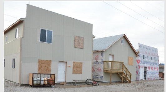
Structural Collapse training prop in initial stages of construction.
